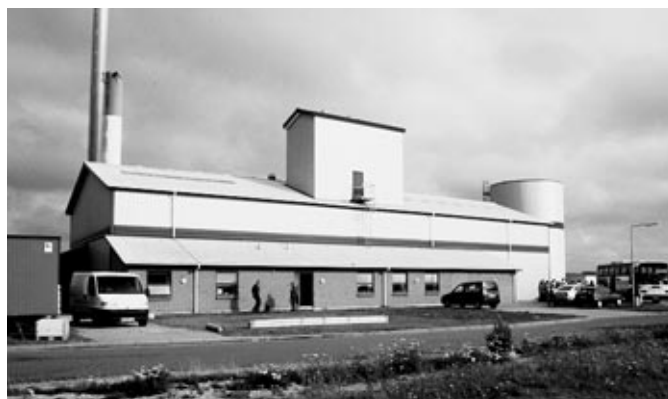
Fig. 5b: Community combined heat and power (CHP) plant, fueled by wood chips, for 300 families in Denmark Photograph by Dr. Donald Aitken
