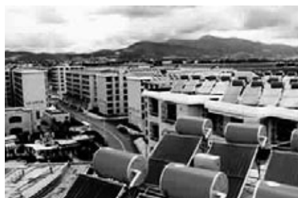
Fig. 13a: Solar Water Heating in China. Source: Li Hua, RENEWABLE ENERGY WORLD , July/August, 2002, p. 105
