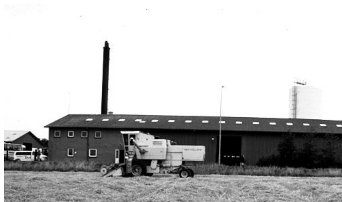
Fig. 6b: Community combined heat and power (CHP) plant, fueled by waste straw grown in the near vicinity, for 300 families in Denmark Photograph by Dr. Donald Aitken
